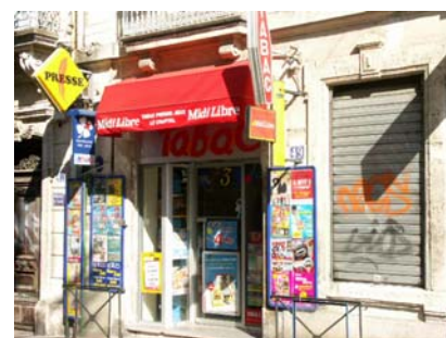
Installation de commerces
